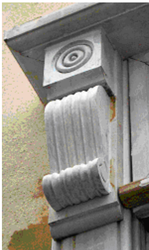
Console under construction Old Bridge
