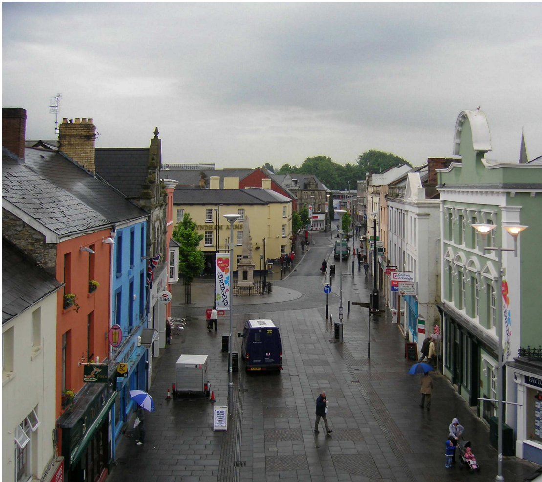
Dunraven Place, Bridgend – Conservation of the heritage buildings maintains local identity, aids sustainability, enhances the prosperity of the town and engenders local pride.
